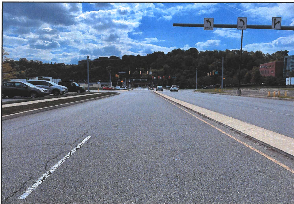
Rear view of a northbound, left turning vehicle from Newbury Drive into the Proposed Site Drive C (stopping sight distance behind)
