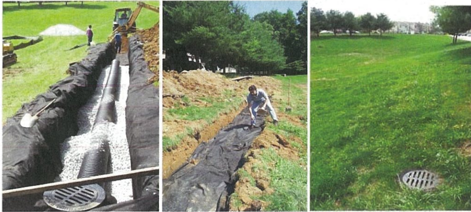
Figure 3: Example of Infiltration Trench Installation
