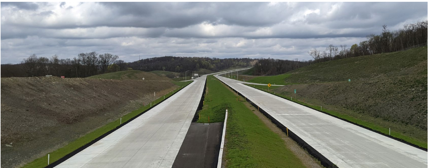
Southern Beltway (Now Open) Under Construction in 2021
