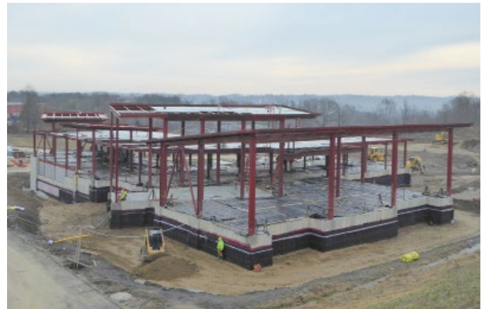
New Municipal Building Under Construction
